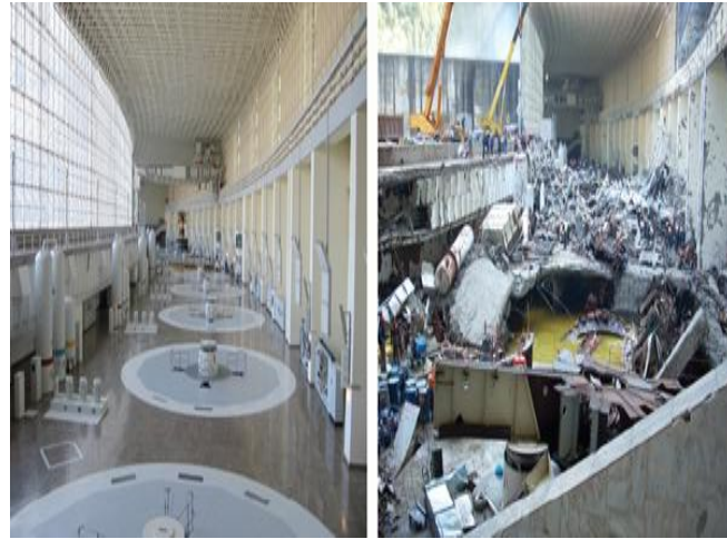
Figure 5. The destruction of the turbine, before and after gallery turbine plant.
