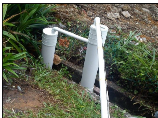
Figure 3 Installed Smart Trap
