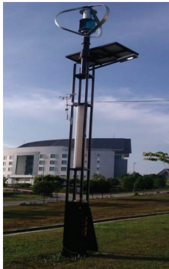
FIGURE 1. Hybrid PV-wind System installed at FKE.
