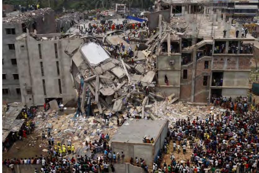
Figure 2.3 Aerial view of the Rana Plaza following the disaster
