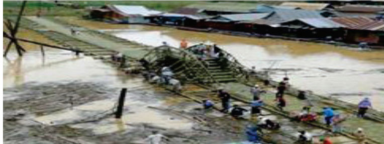
FIGURE 8. Bamboo floating raft bridge under construction (Svamivastu, 2013)
