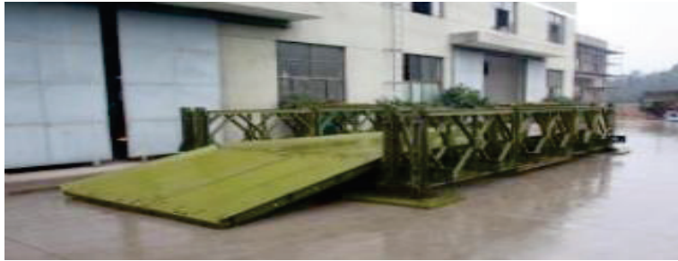
FIGURE 1. Installation of compact 100 Bailey bridge (Azrul & Norazman, 2016).
