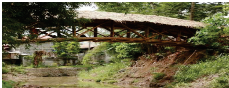
FIGURE 9. Side view of Matina bridge (Fitrianto, 2010)
