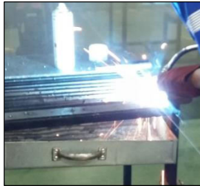
Figure-6. Welding process.
