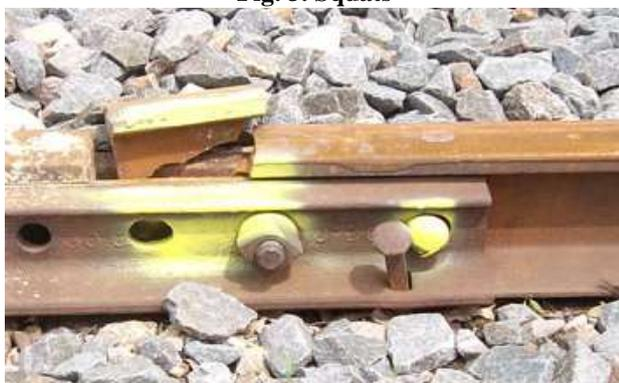
Fig. 4. Broken end rail
