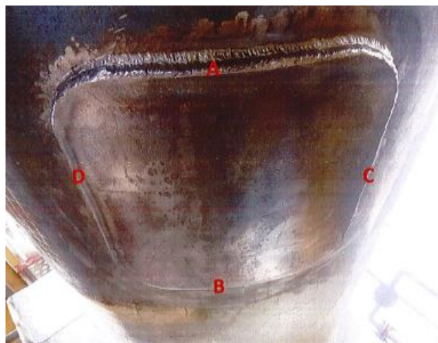
Figure 8. Location for Hardness Test after Fillet Weld.
