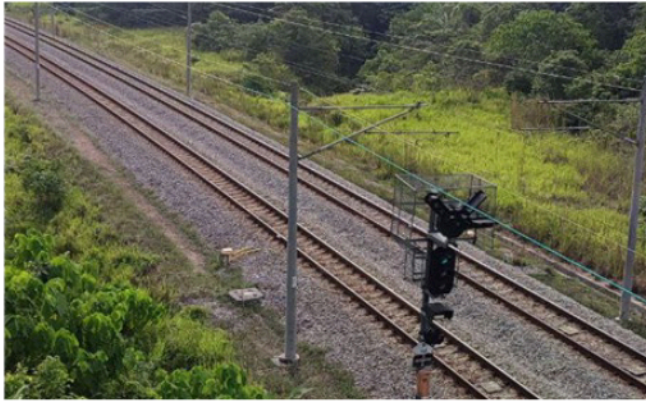
Fig. 1. Simple overhead catenary
