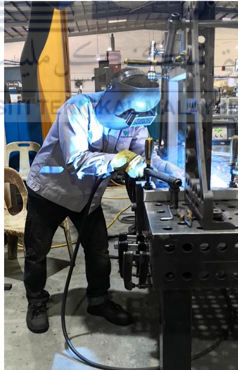
Figure 4.1: Welder rotates his body to achieve welding angle
