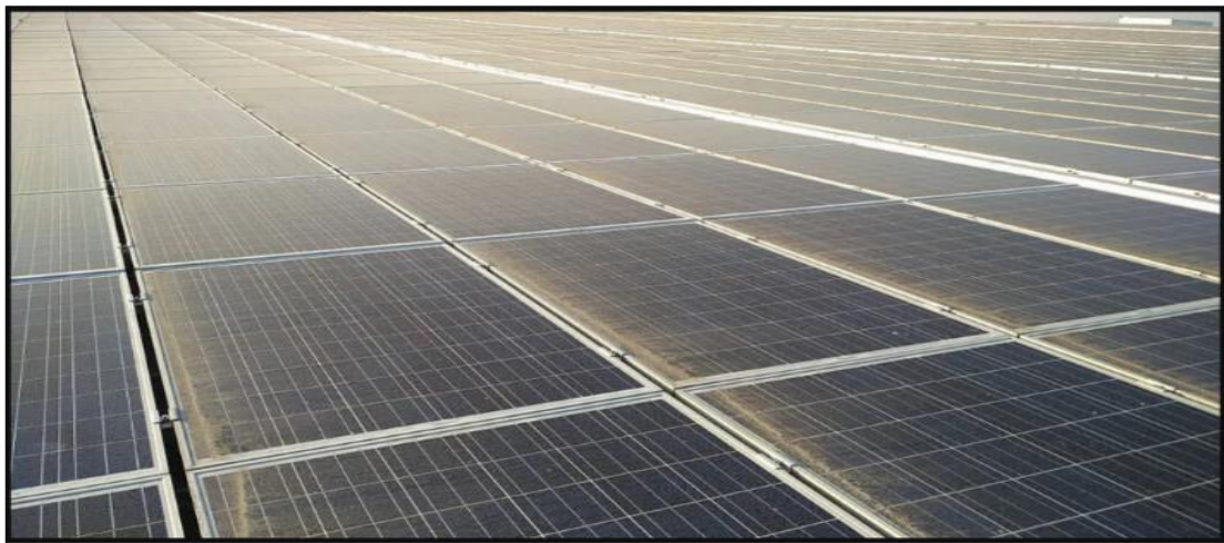
Fig. 8. Dust on solar panel [50]
