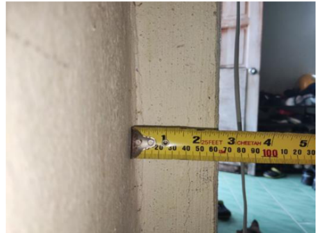
Figure 15 Measurement of Fixed Wall Depth.
