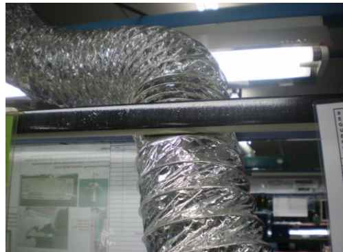
Photo 2: Flexible ducting was dented.
